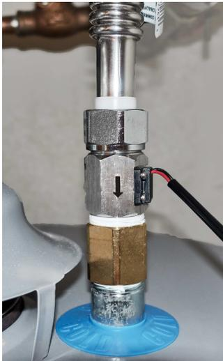
9. Connect the flow meter to the wiring harness via the JST connector ensuring it snaps together securely.
