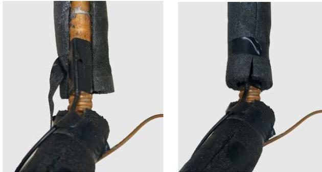
11. Place the other temperature sensor against the hot water outlet pipe of the water heater and tape it securely in place.
