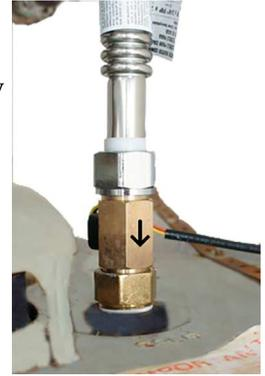
9. Place the temperature sensor against the hot water outlet pipe of the water heater and tape it securely in place. Note: The temperature sensor must be taped securely in place **UNDERNEATH** the insulation that is covering the pipe.
